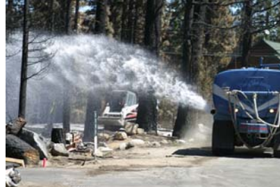
Wetted debris during clean up of 2003 Angora wildfire
