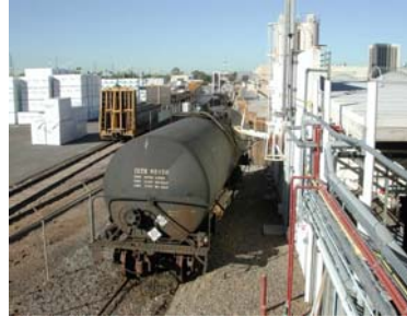
DPC chlorine release
