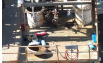
Destroyed filter housing at BP refinery
