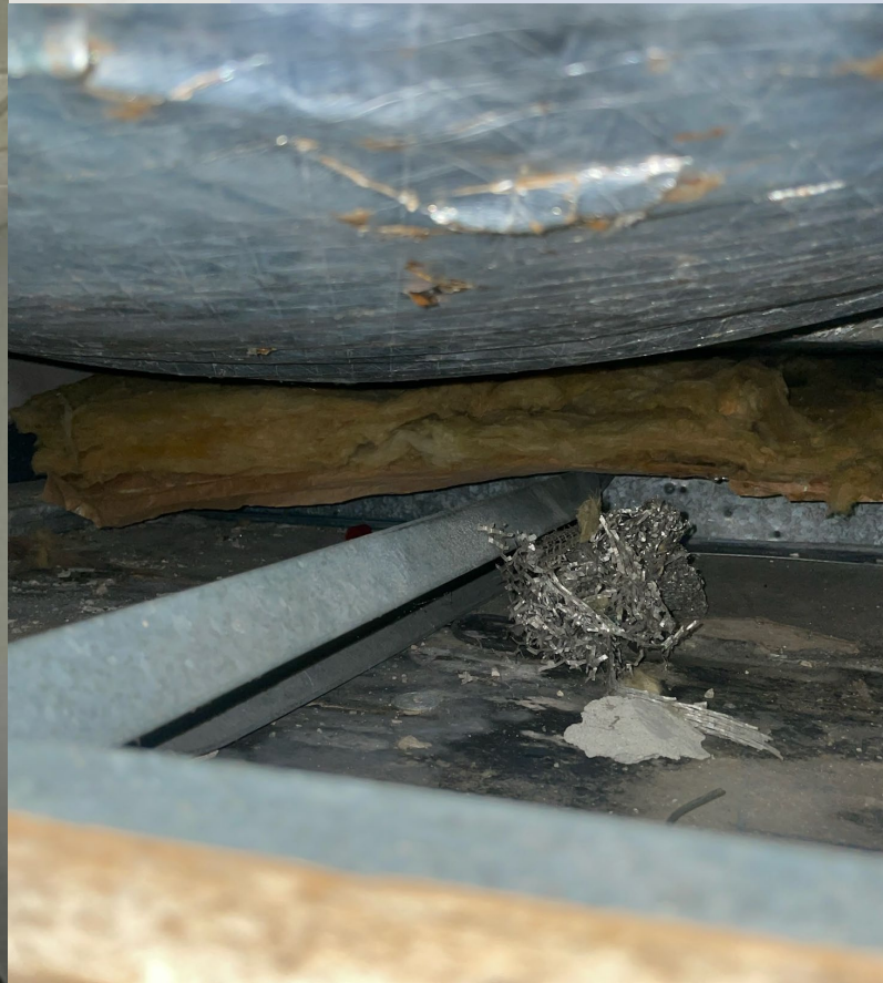
Stachybotrys growth on top side of ceiling
