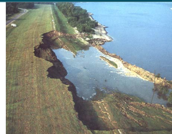
Picture of levee breach
