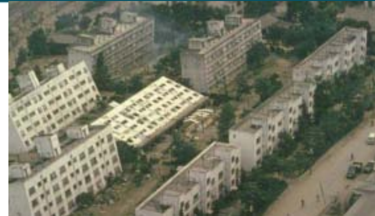
Liquefaction results after earthquake in Japan
