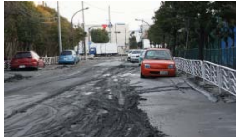
Liquefaction from 2011 Japan earthquake
