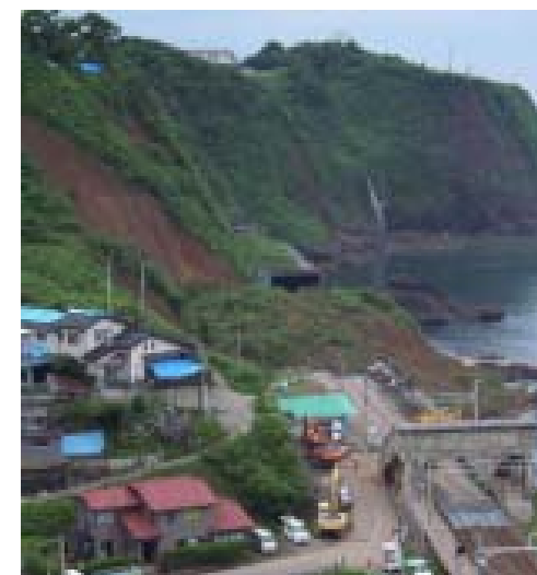
Landslide Oumigawa Japan 2007
